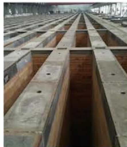
碳素焙烧炉 Carbon Baking Furnace
