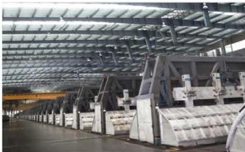
电解槽 Electrolysis Workshop
